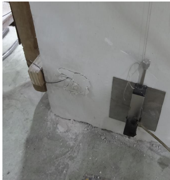
Photograph 7.1.2.1. Damages associated to the compressive loading.
