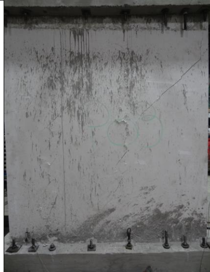
Photograph 7.2.2.3. Typical shear failure in test sample HL-UO-03. Diagonal cracks are observed.
